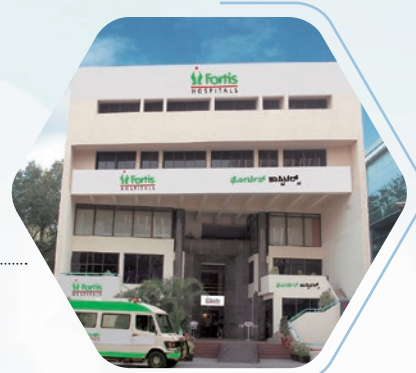
Fortis Hospital, C.G. Road Bengaluru
