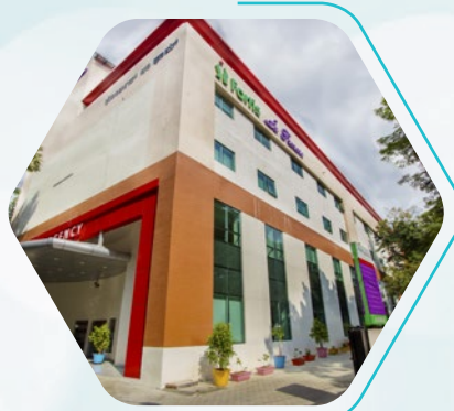
Fortis Hospital, Richmond Road Bengaluru
